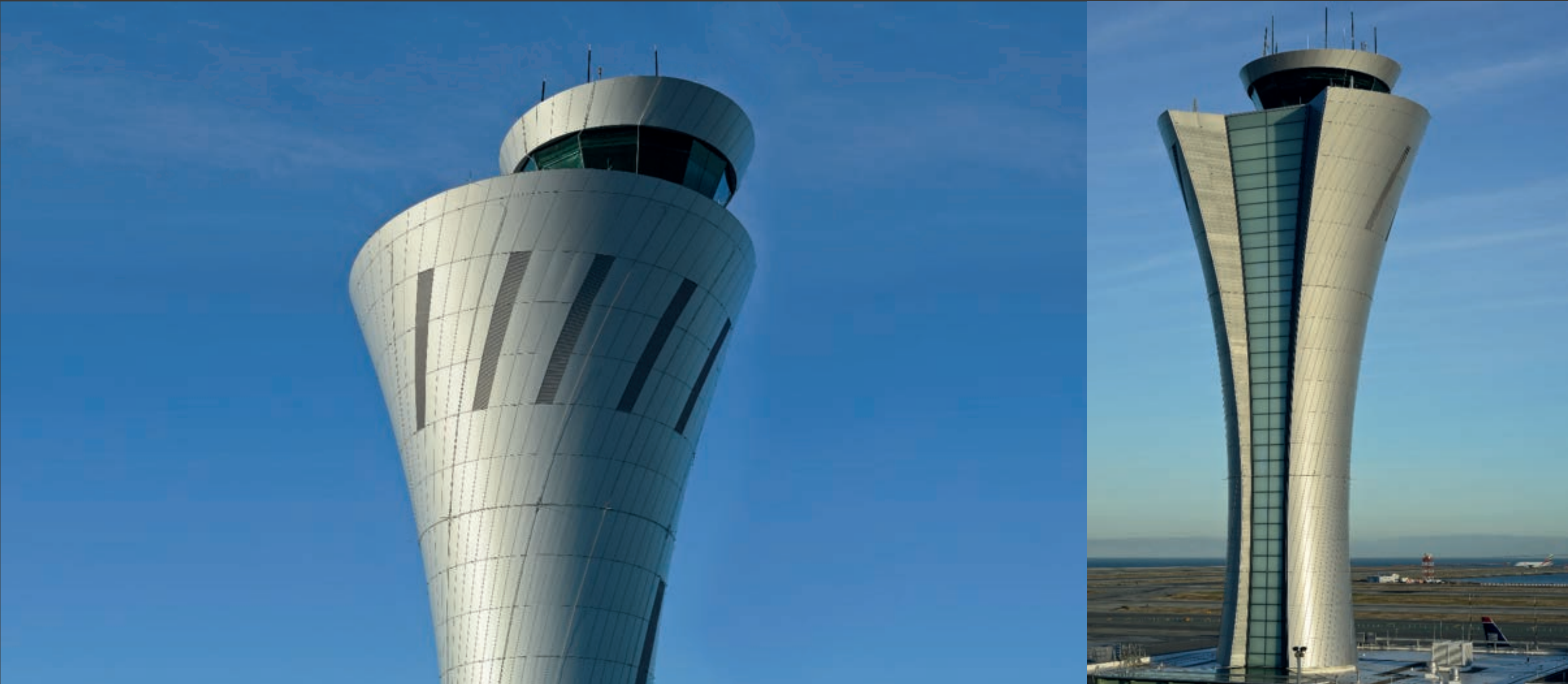
Air traffic control tower | San Francisco | U.S.A
